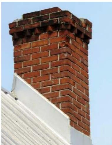
Photo 28 – North chimney showing brick and mortar deterioration on the south and east sides.
