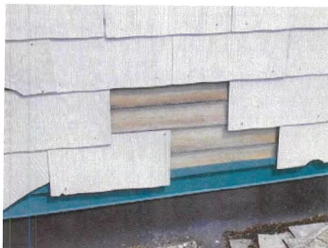
Photo 31 – Wood siding under the asbestos tile siding of the church. The area shown is at the south end of the church.
